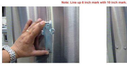
Step 3: Use bracket center hole to align with cross mark. Note: Use pencil/marker to mark hole pattern.
